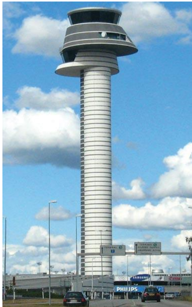
Fig. 1 Arlanda Airport Control Tower, Stockholm, Sweden
