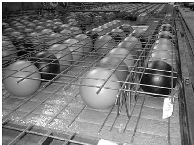
Fig. 8 Bubble decks produced with powder type SCC with Fly-ash
