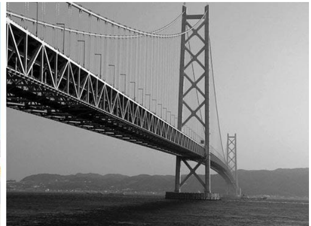
Fig. 3 The Akashi-Kaikyo Bridge, Japan
