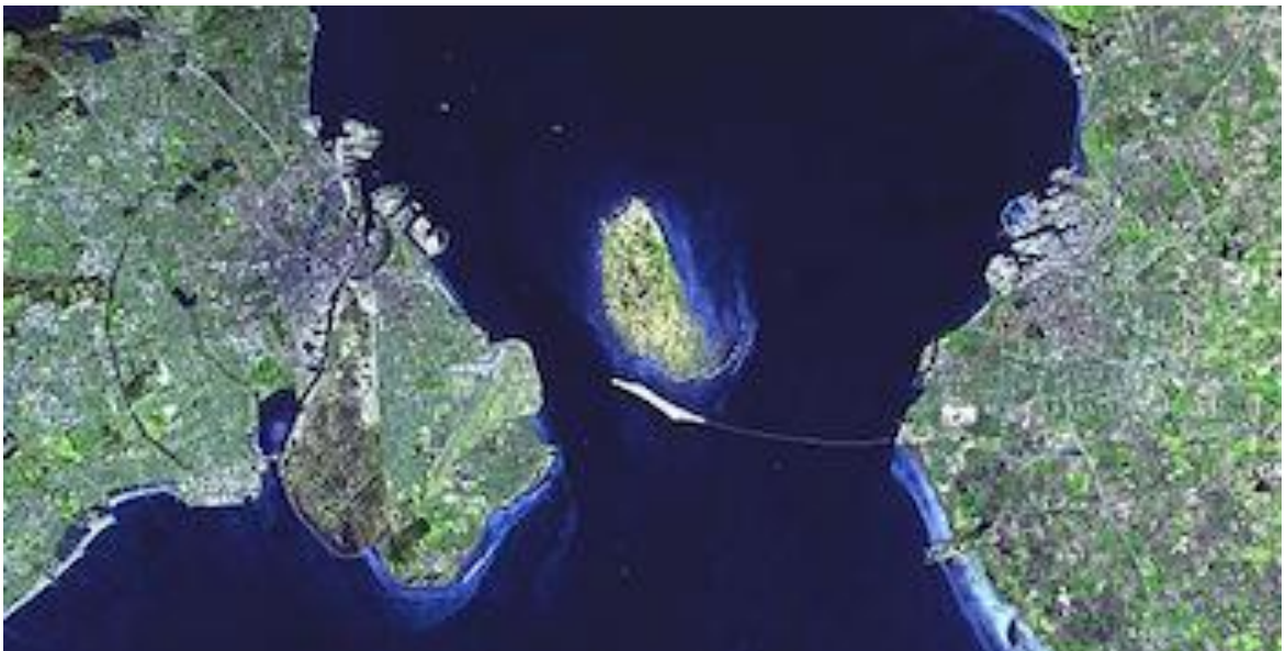
Aerial view showing the Oresund Bridge. Denmark in on the left and Sweden in on the right. The visible white arc in the middle of the water is Peberholm, the artificial island
