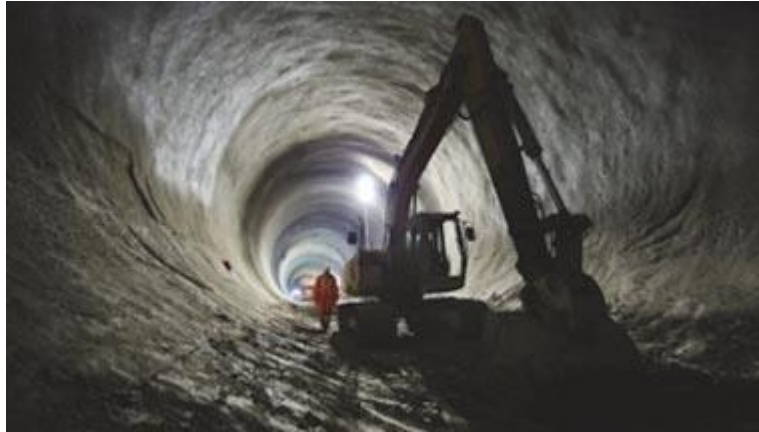
Fig. 4 Tunnel Lining construction in Japan
