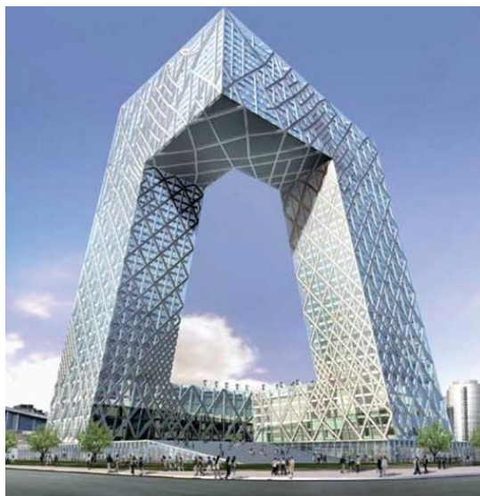
Fig.6 CCTV New Station, Beijing
