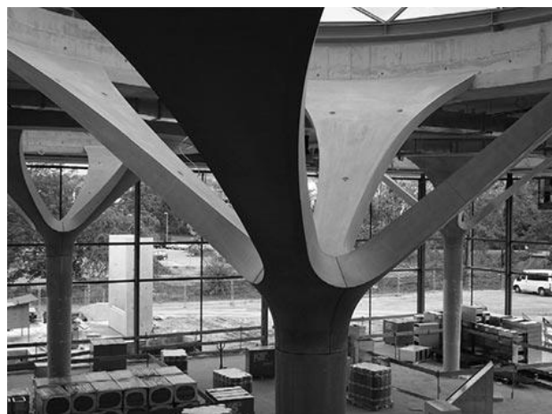
Fig. 7 Complex column made using SCC
