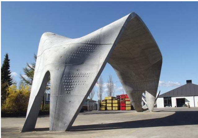
Fig. 2 PASCHAL plant premises in Aarhus
